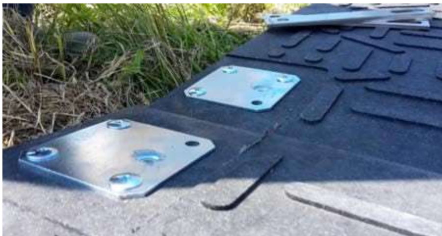
1. Adjacent mats installed ready for connection.
